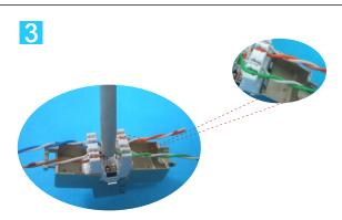
Follow the wiring sticker to place the wires into IDC slot. Keep the pairs twisted as possible as you can.
